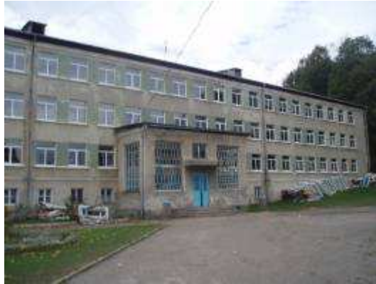
New windows were installed
