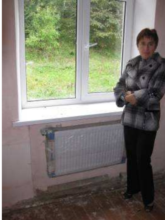
New heating system was installed by the state. We replaced the windows
