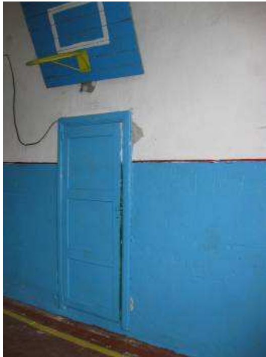
Door to supply room
